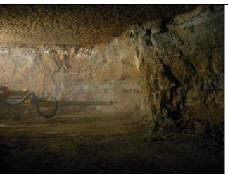
Figure 6. Face fall after undercutting layer C.
