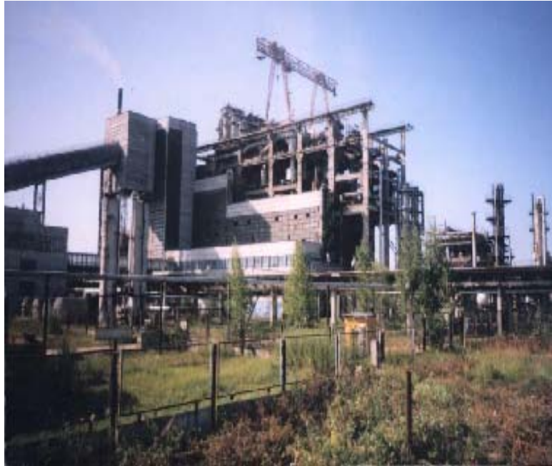
Oil Factory in Narva, Estonia, built under ATOMENERGOPROEKT's design, 1980-84
