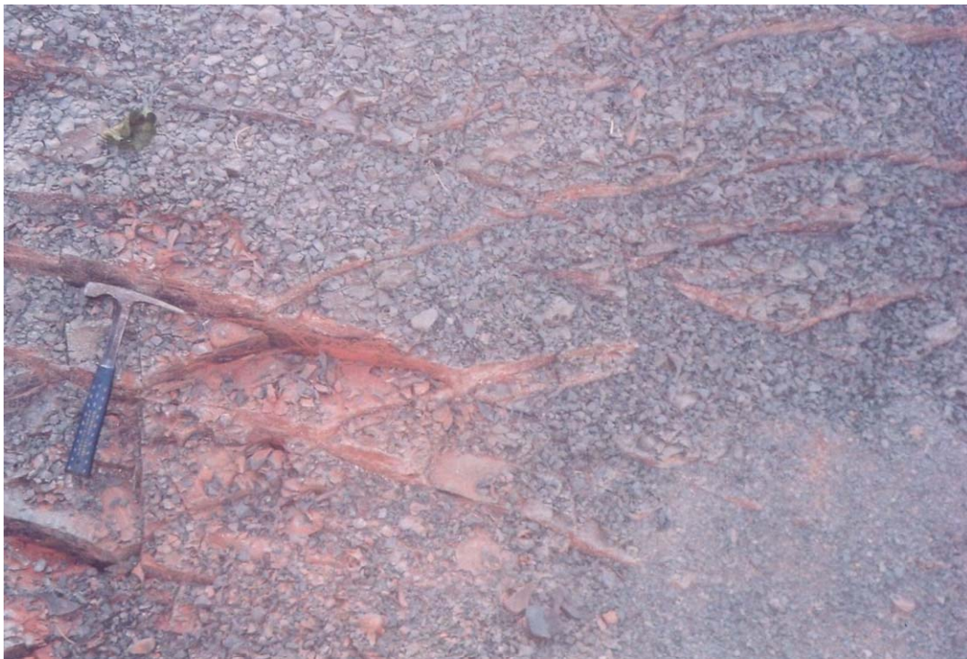
Figure 5 Regular fractures trending \text{N}30^{\circ}\text{W} dipping 80^{\circ}\text{E} and \text{N}70^{\circ}\text{E} dipping 75^{\circ}\text{NW} on the Edaga Arbi shale.
